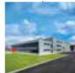
Site Feluy INSULATION
